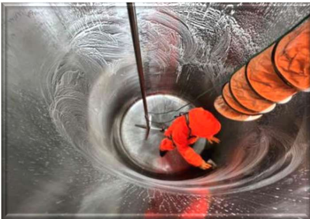
Cleaning inside tank
