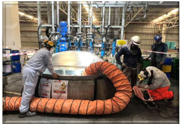
Cleaning inside tank
