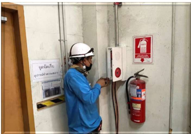
Checking the fire alarm system
