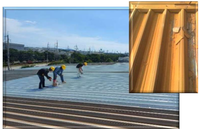
Repainting on a roof
